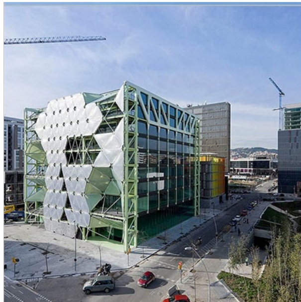
Figure 44. MEDIA-TIC, Architects: Enric Ruiz Geli, Location: Barcelona, Spain, Completion Year: 2009, Credits: archdaily.com, © Stijn Bollaert
