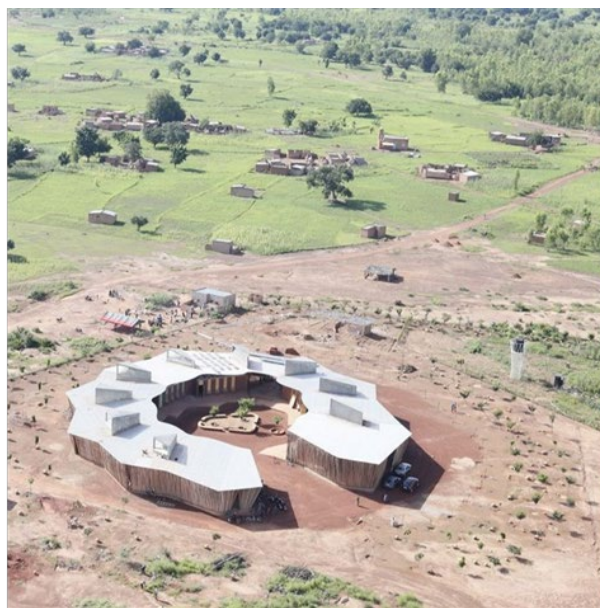
Figure 38. LYCEE SCHORGE SECONDARY SCHOOL, Architects: Kéré Architecture, Location: Burkina Faso, Completion Year: 2016, Credits: archdaily.com, © Iwan Baan
